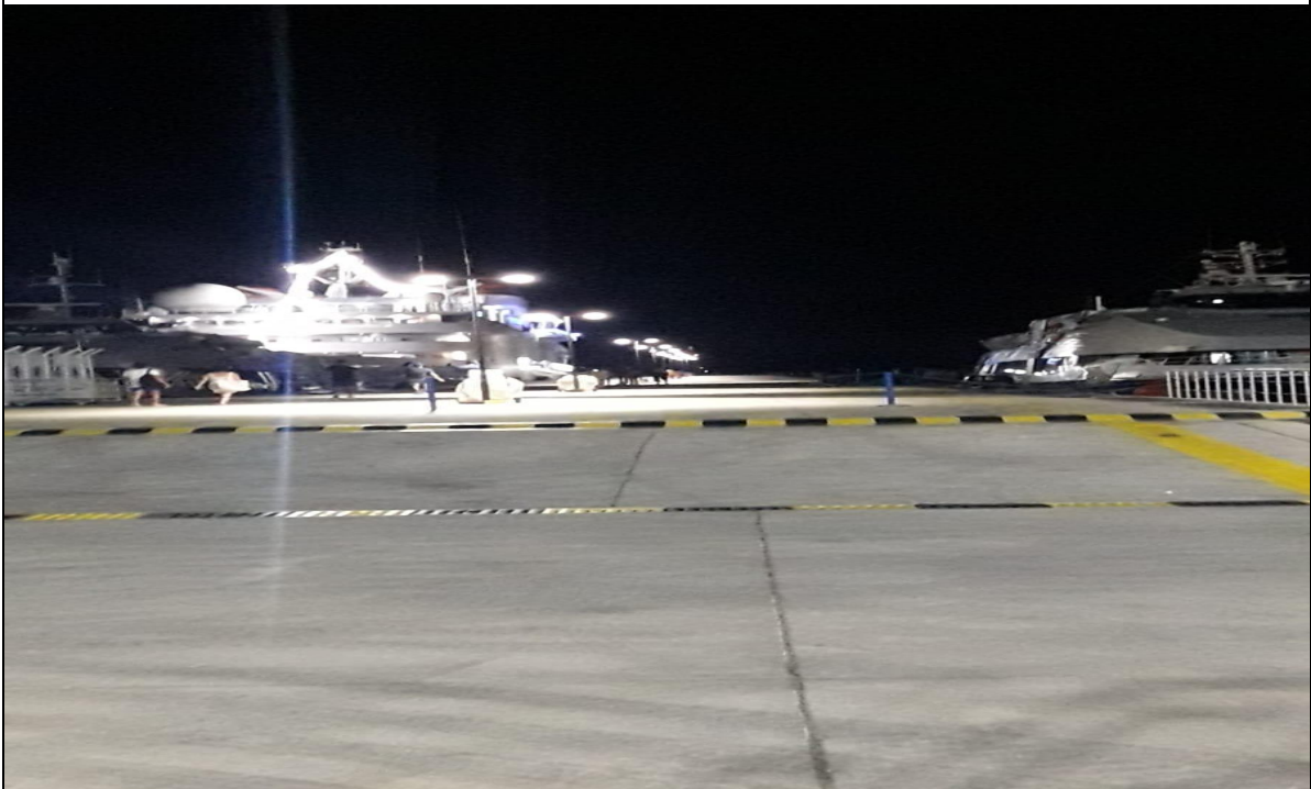
Figure 6 Led lighting on the pier
