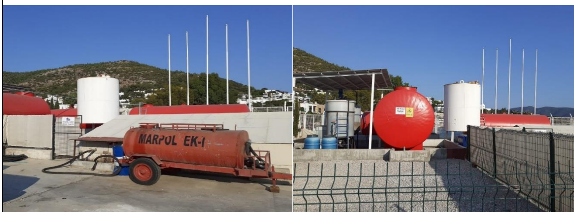
Figure 5 Waste Reception Facility and Waste Reception Truck
